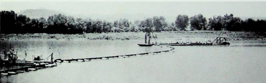
The Dredge cleaning the river.
