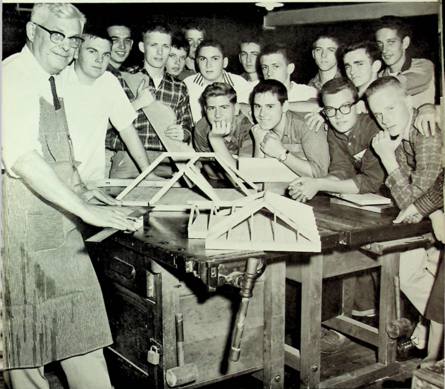
Mr. Multer Explains The Basic Principles Of Roof Framing To His Woodshop Class
