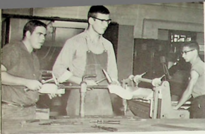
David Gray, David Martin, and Tom Beard work on a project in Sheet Metal Shop under the supervision of Mr. Goings, instructor.
