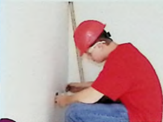
Judd Evans skillfully adds a new outlet to a wall.
