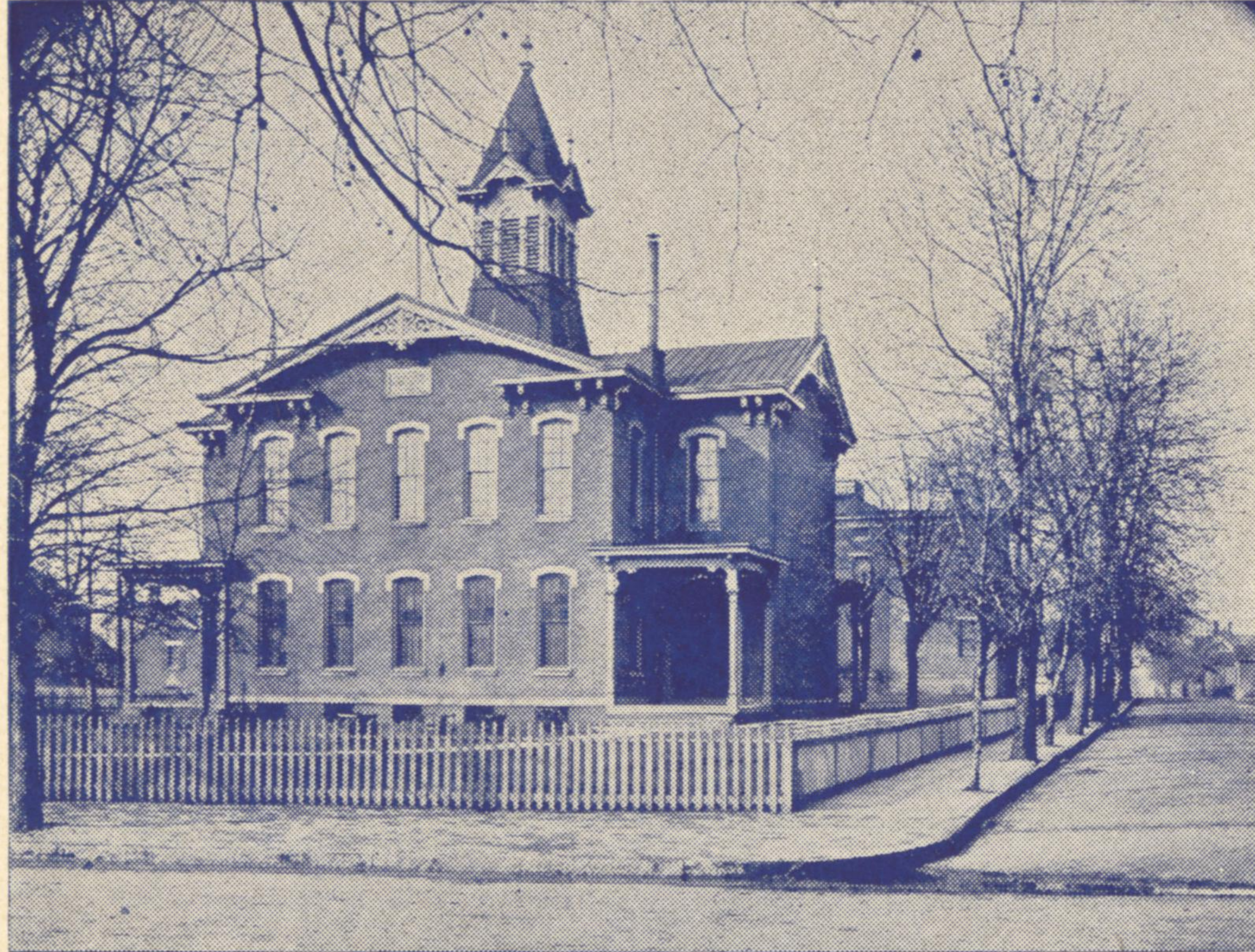
THE OLD HIGH SCHOOL BUILDING.
