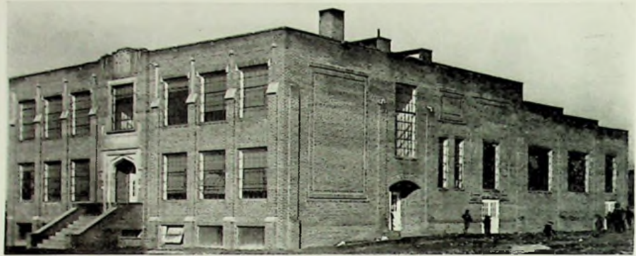
SOUTH WEBSTER GRADE BUILDING
