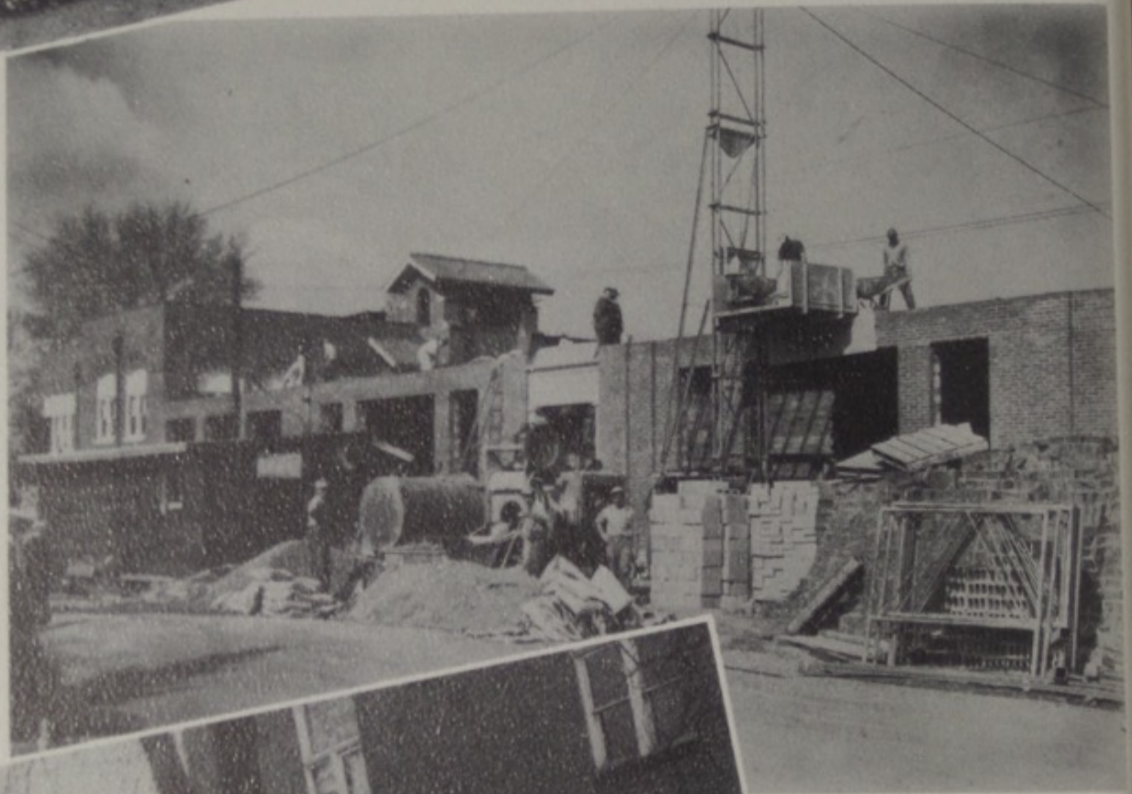
Construction underway on the new Valley grade building in Lucasville.
