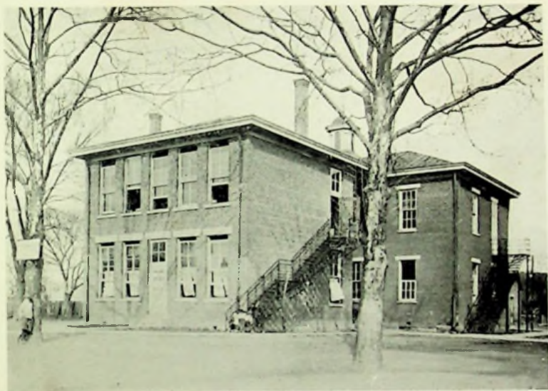
"THE OLD BUILDING"
