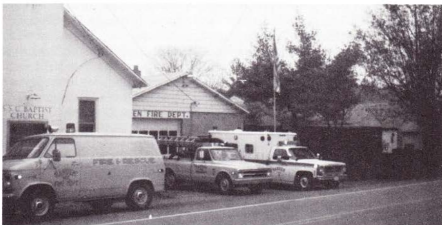
Fire Department Front
