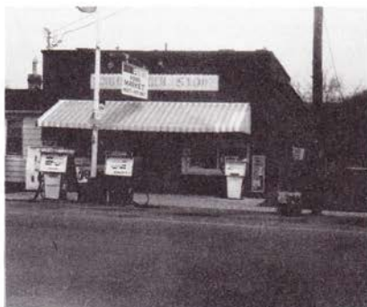
Brick store built in middle 1920's
