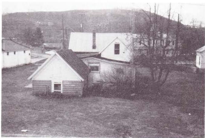
Looking south to Dunlap and Hoffer Hill former South Store and residence from rear.
