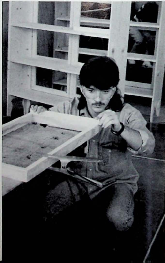
Joe Ayers installs floor joists on his model house. This was an interesting project for the students.
