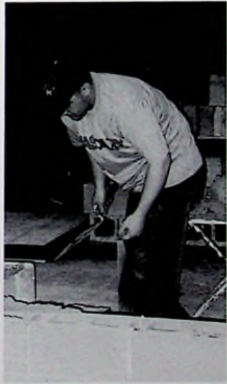
Derick Blanton slaps cement on the blocks before adding another. He was in Masonry class.
