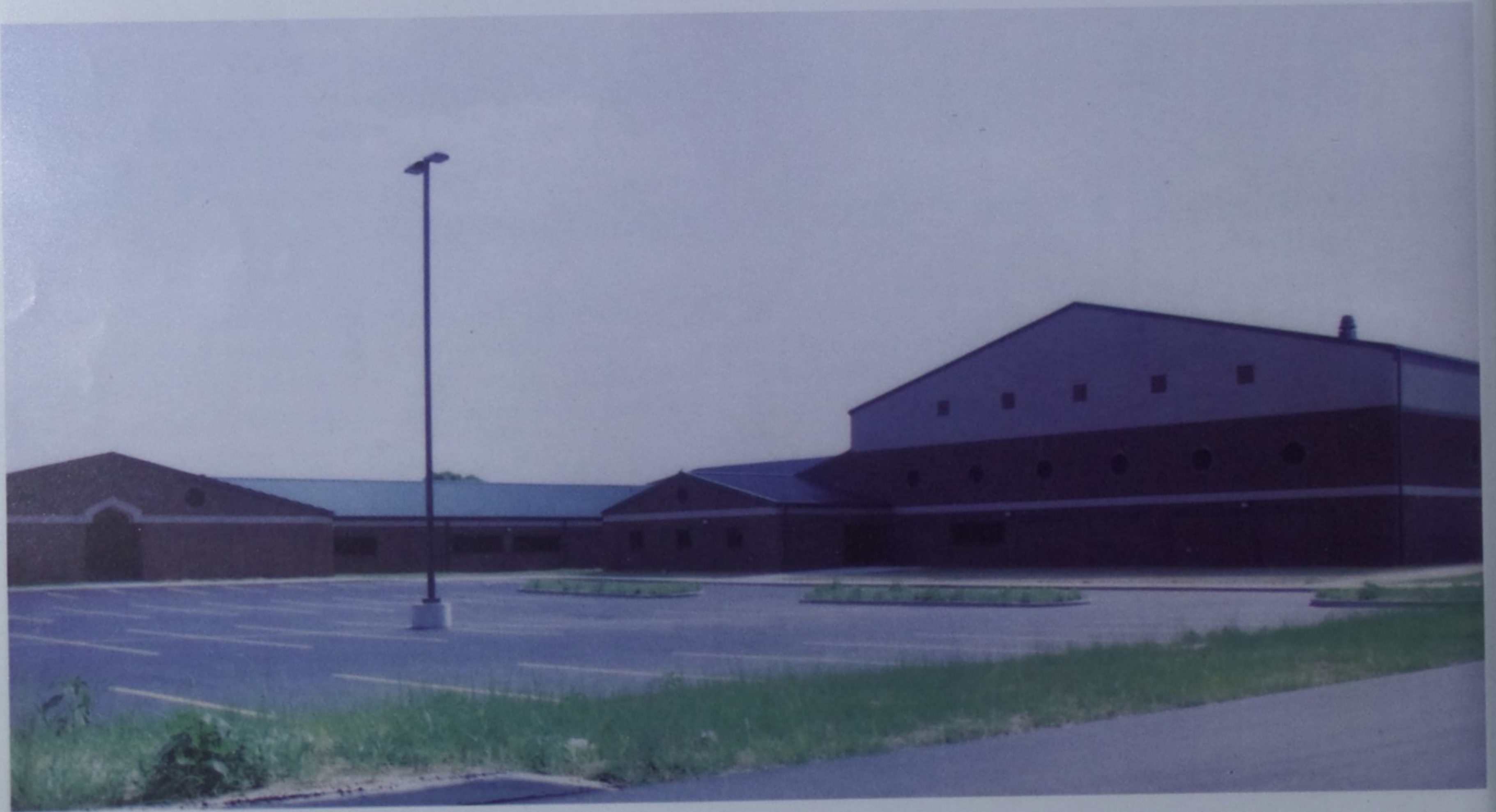
E ast view of high school including gymnasium.
