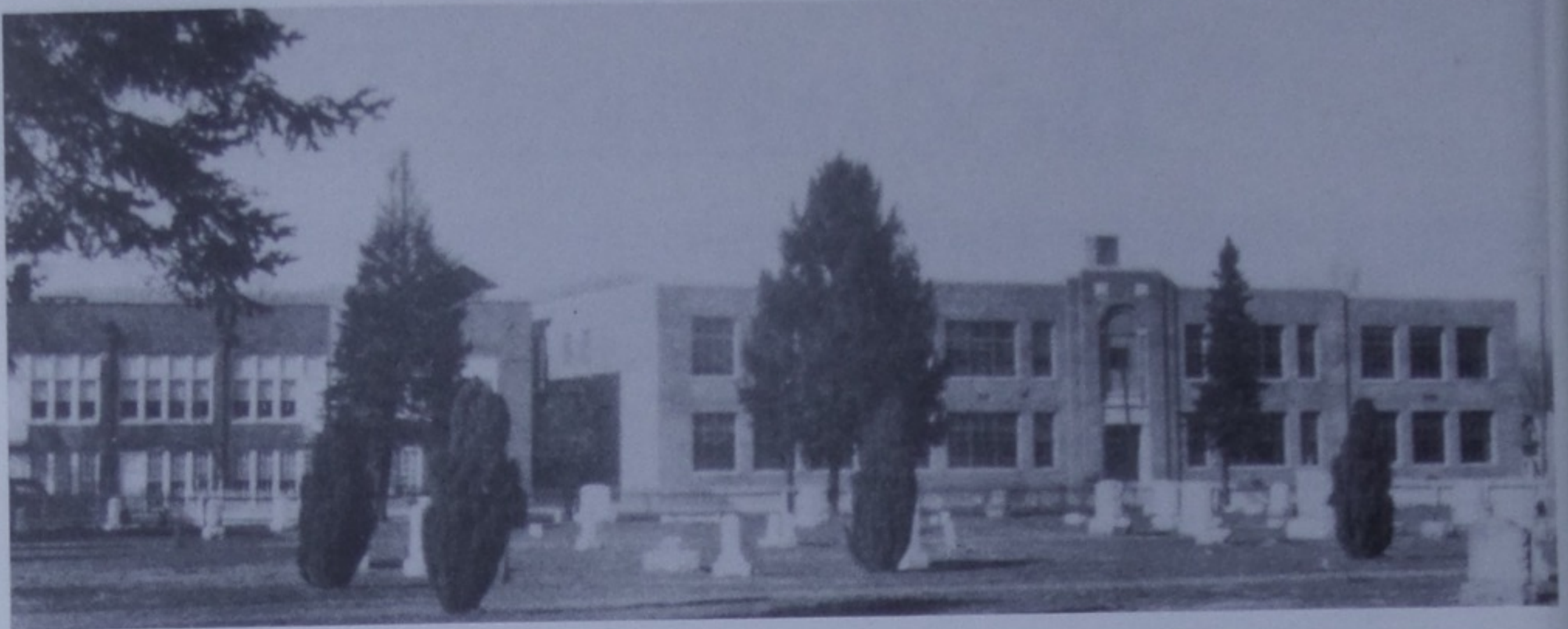
Former Valley Elementary. This building was built in 1911 and once served as Valley High School.
