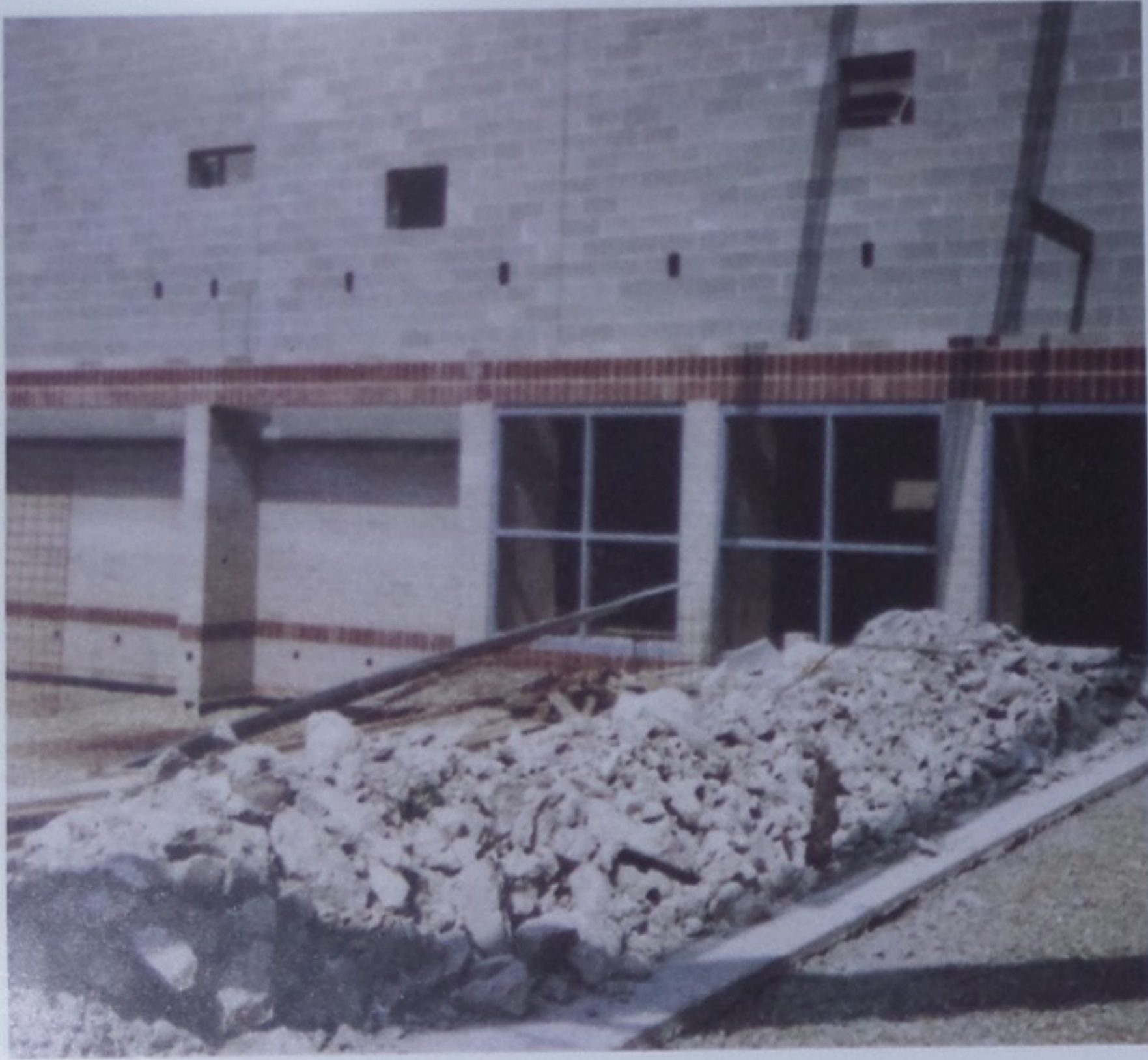
A view of the high school cafeteria area while under construction.
