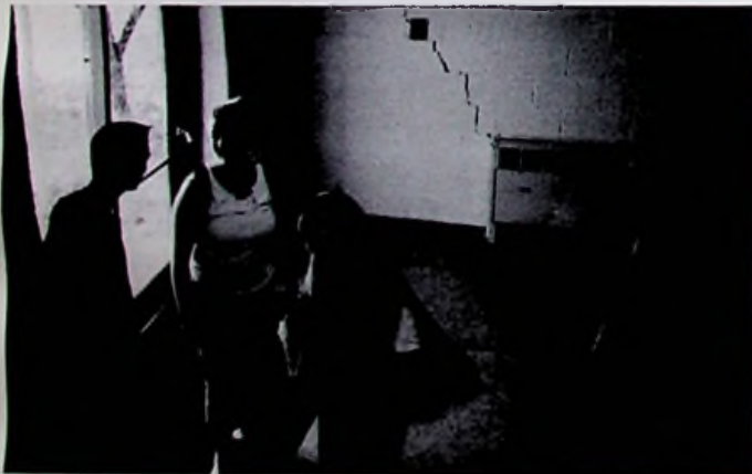
Leaving the cracks behind.
