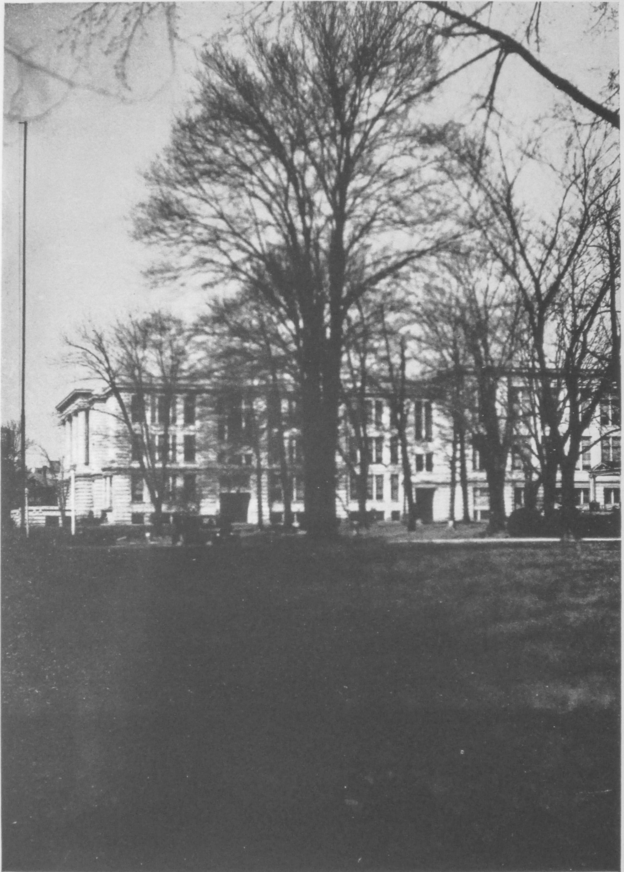
APPROACHING FROM THE EAST
