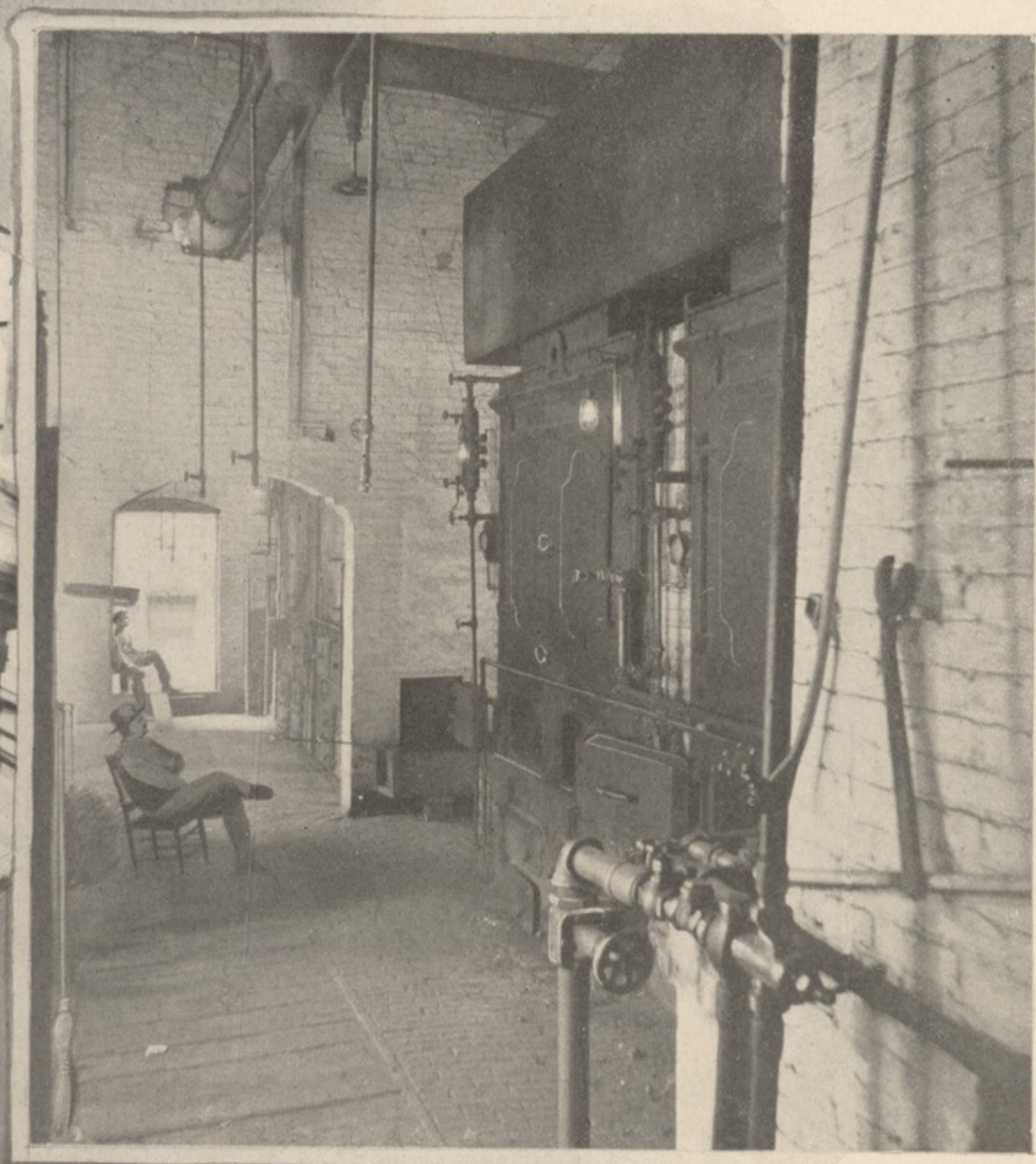
F OUR BOILERS, capable of developing 700 horse power, feed the engines. They are all fitted with down-draft smoke-consuming furnaces which work so perfectly that scarcely any smoke is ever discernable coming from the stacks. The other view on this page shows the men at work setting up the cases.
