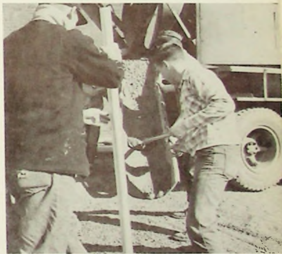
The field's fence is erected.
